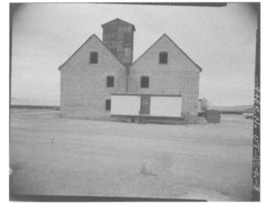
View of southwest end of German Village looking northeast. Courtesy Library of Congress, Historic American Engineering Record, Historic American Building Survey.
